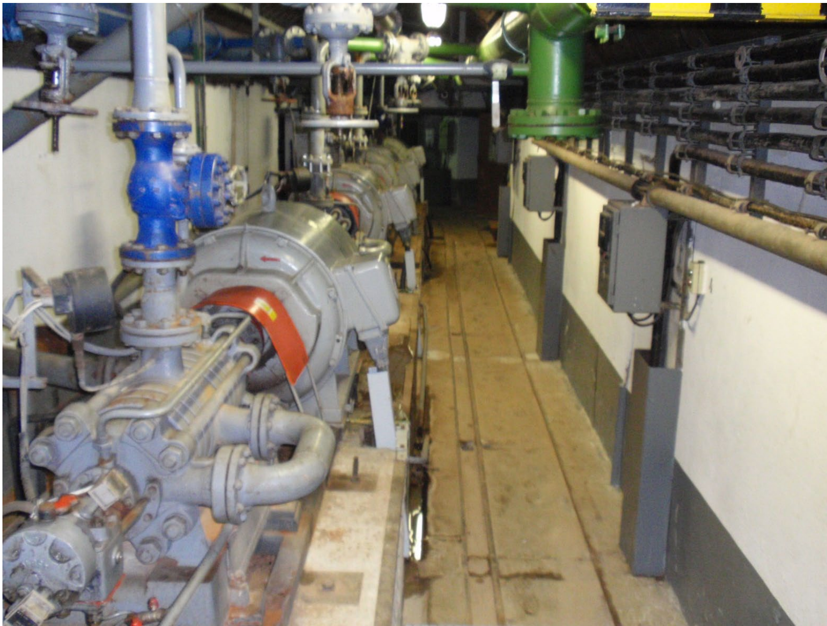
Fig. 6S. Pumps that draw water from depths exceeding 500 meters for use in the spa (photographed by the author T.Ř.).
